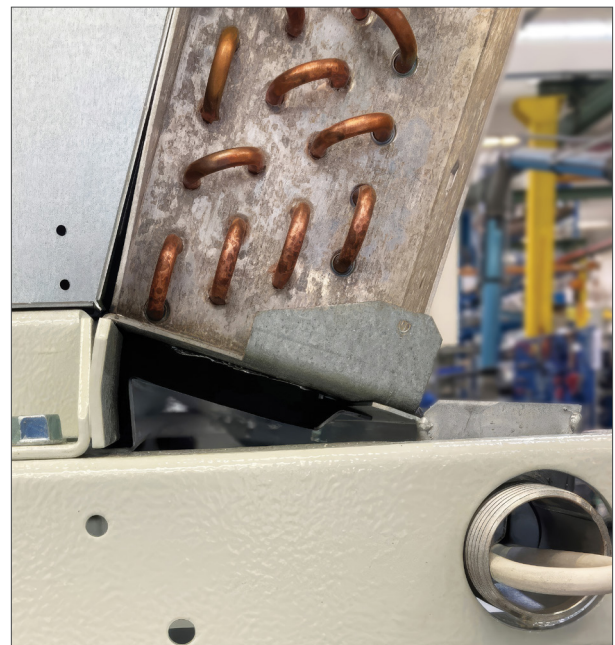
Figure 2.6 | Heat Traced Drain Pans and Coils
