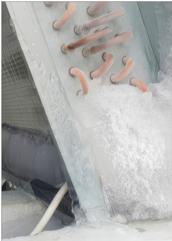
Figure 2.1 | Frost on Refrigerant-to-Air Coil
