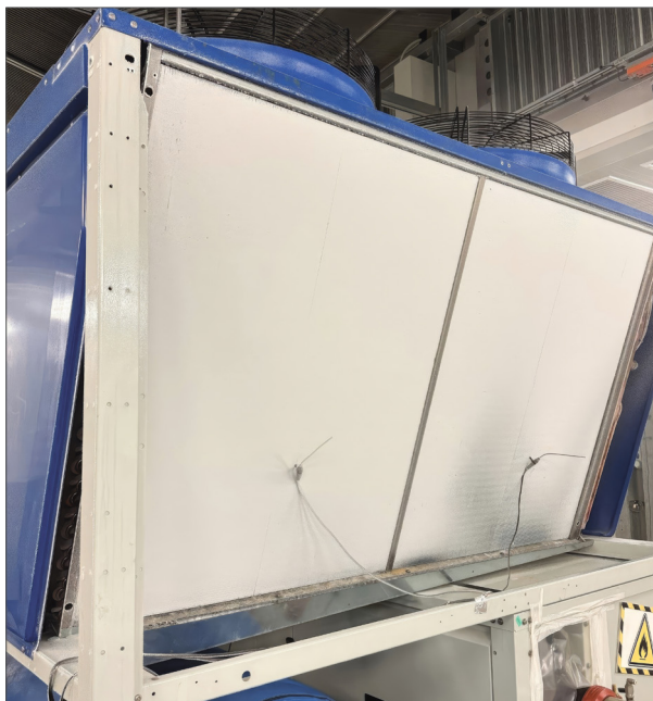
Figure 2.5 | Sloped Drain Pans
