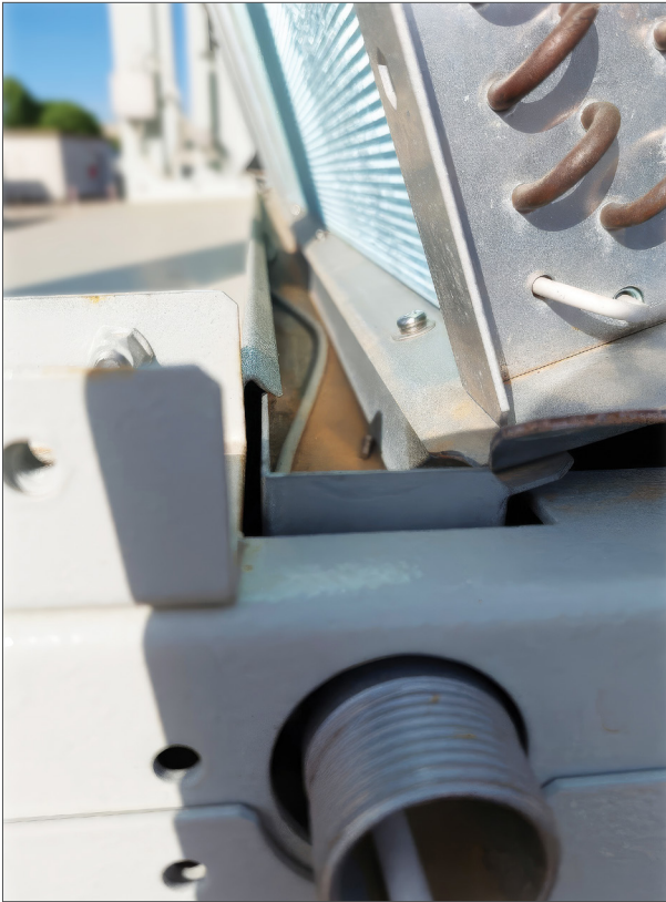
Figure 2.7 | Heat Traced Down Pipes
